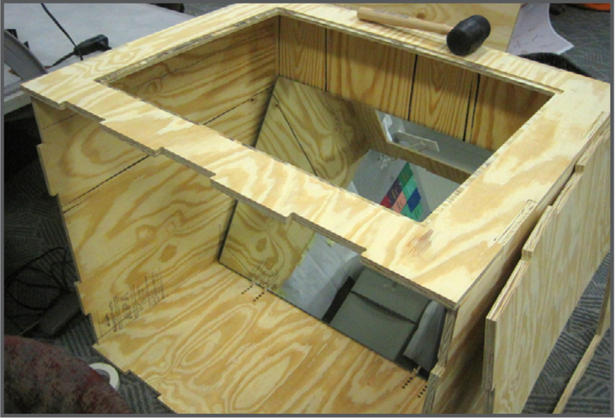
Figure 4. A view of the table as it was being constructed.
